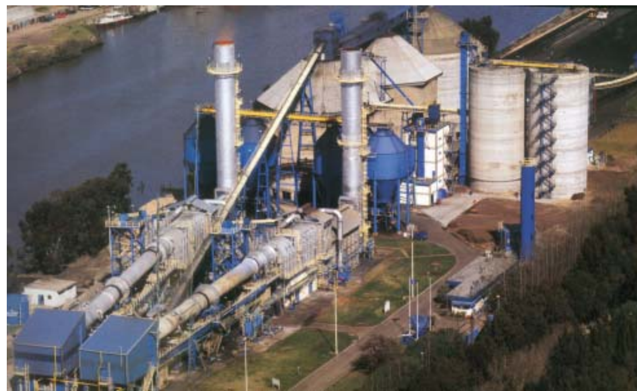
Copetro S.A. Plant, La Plata Port, Ensenada Province of Buenos Aires, Argentina
